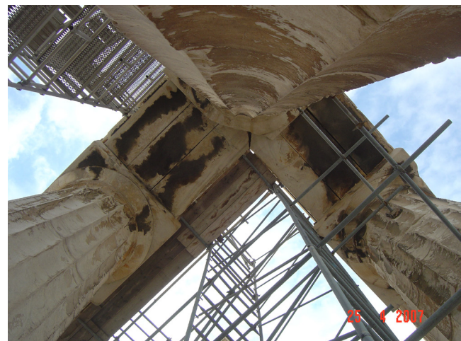
Fig. 14. Parthenon. Northwest corner: Structural problems on the architraves of the north corner. View from west (photo S.Gesafidis 2007).
