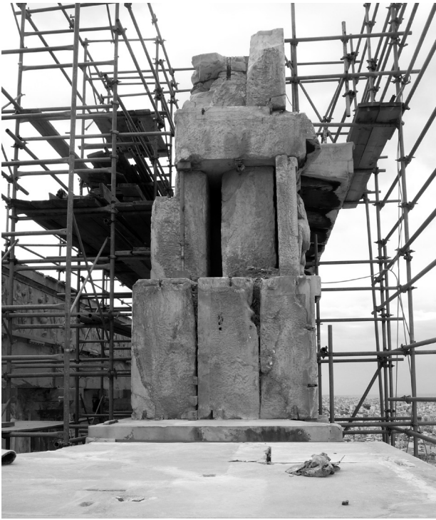
Fig. 19. Parthenon. West pediment: Structural problems due to the action of the metal clamps in combination with the quality of the marble and, in addition, to the movements caused by seismic activity (photo T. Souvlakis 2012).
