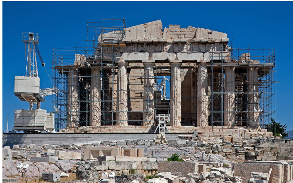
Fig. 18. Parthenon. Current restoration works at the two corners of the entablature of the west side. View from northwest (photo T. Souvlakis 2012).
