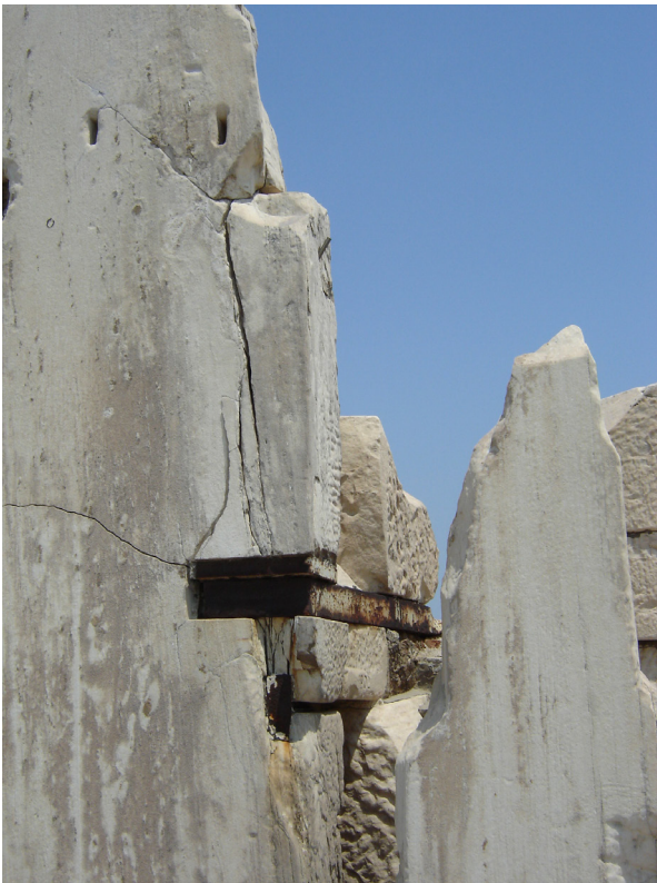
Fig. 13. Parthenon. West side. Exterior iron joining elements by the earlier interventions on the Acropolis monuments (photo V. Eleftheriou 2007).
