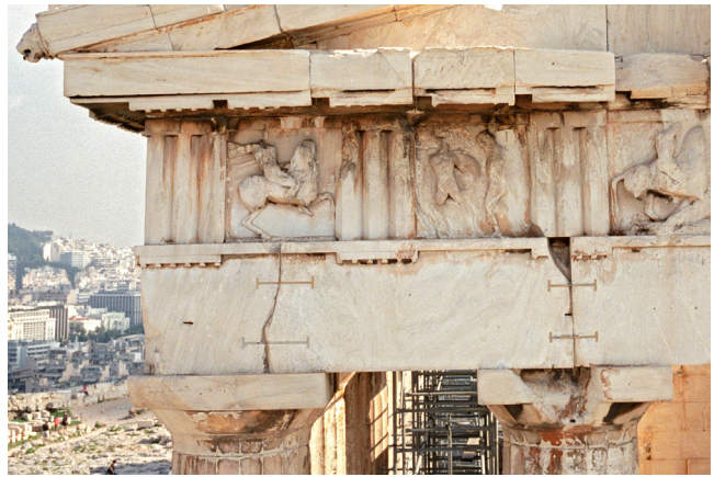
Fig. 14. Parthenon. Northwest corner: Structural problems on the architraves of the north corner. View from west (photo S.Gesafidis 2007).
