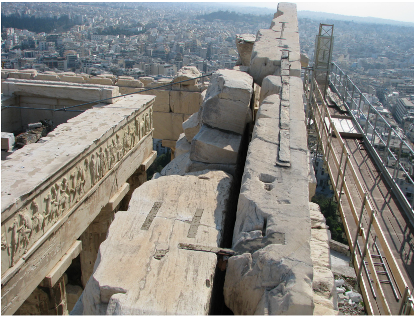
Fig. 11. Parthenon, the upper part of the west pediment. Mechanical damage. Fractures due to the expansion and oxidation (rusting) of the iron dowels used in earlier restorations. View from north (photo V. Eleftheriou, 2008).
