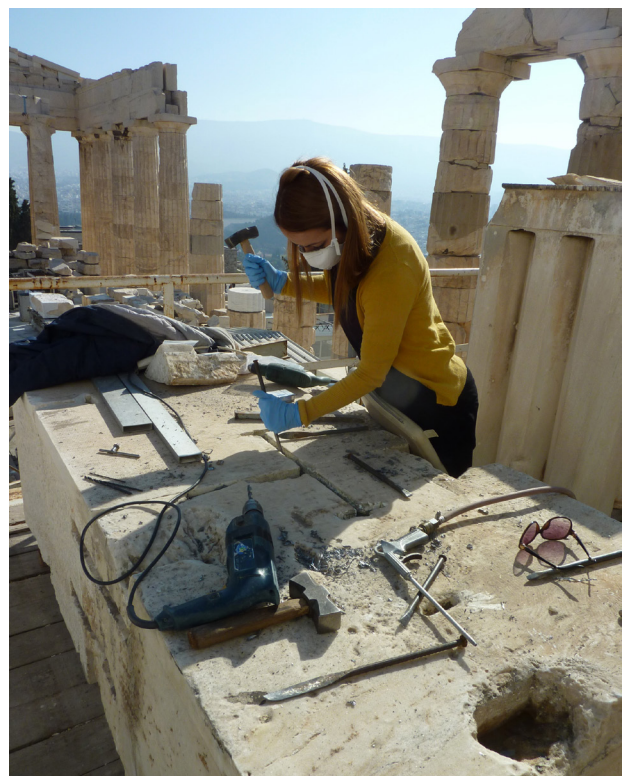
Fig. 3. Removal of rusted iron reinforcements from the blocks of the Parthenon (photo Christodouloupoulou 2012).
