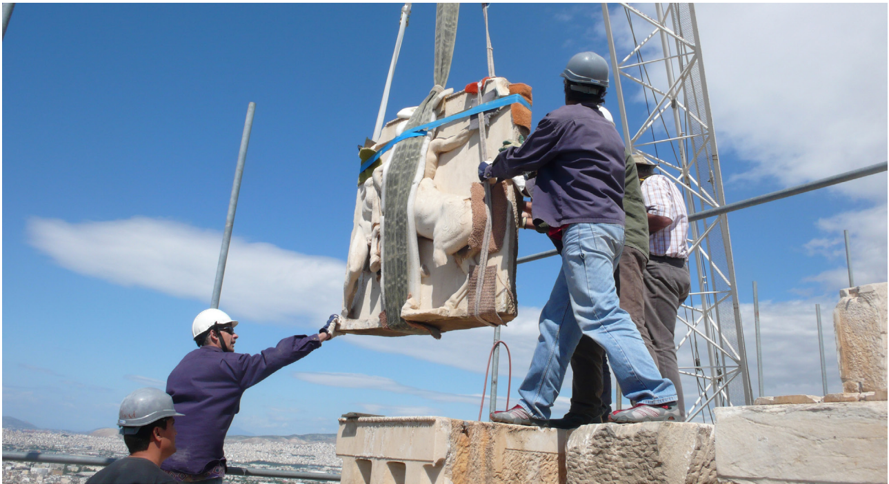
Fig. 2. Dismantling the blocks of the west side of the Parthenon (photo V. Eleftheriou, 2012).
