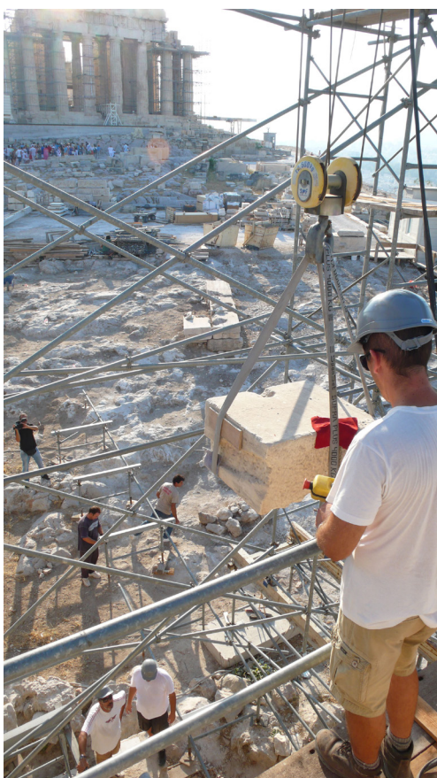
Fig. 4. Propylaea after completion of the restoration of the southeast corner. Two wall blocks and a crown block made in new marble have been completed (photo V. Eleftheriou, 2012).
