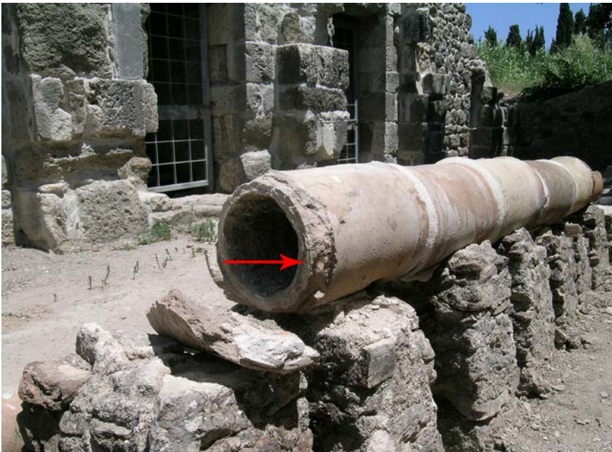
Fig. 11. Kos, clay pipes along the street south of the Odeion: observe the calcareous incrustations inside, which are about 2 cm thick and are indicated by a red arrow (photo G. Rocco).
