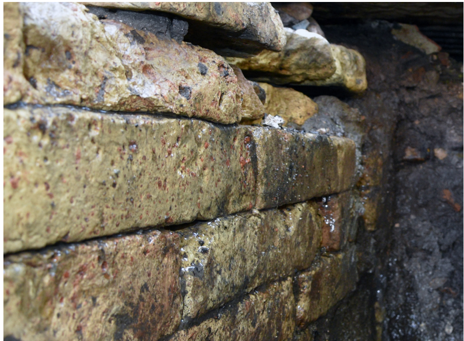
Fig. 4. Aquileia, area of the Roman theatre: groundwater emphasizes the presence of abundant chamotte (reddish inclusions) in the bricks of a major drain, 1 st c. BC-1 st c. AD (photo by the author).
