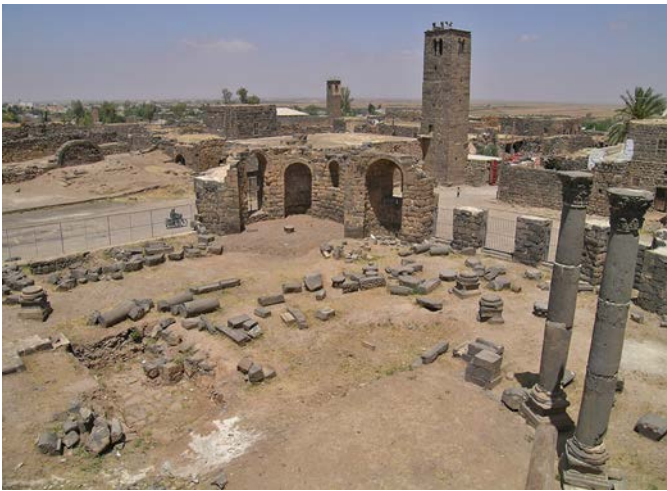
Fig. 7. Bosra, Church of SS. Sergius, Bacchus and Leontius. The position of the nave after the latest conservation work in 2004 (photo by the Author).
