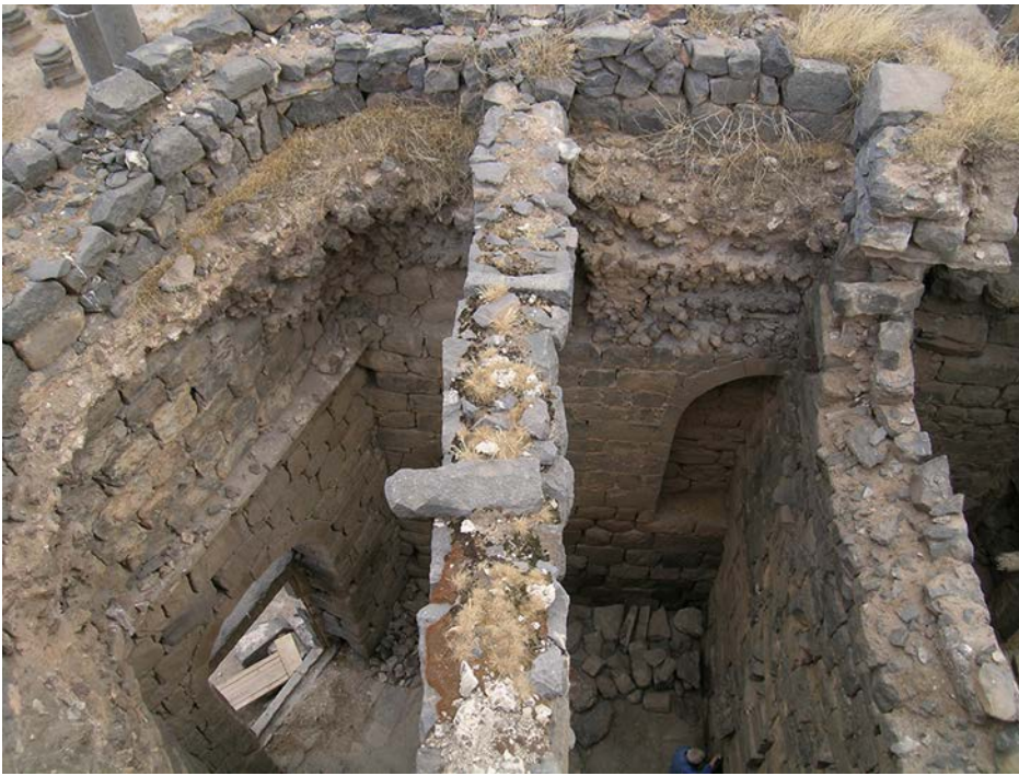
Fig. 9. Bosra, church of SS. Sergius, Bacchus and Leontius. Chamber 'b' from above, showing the remains of the vault, set on the cornice of the central body and on the recess of the northern wall. The chamber is divided by partitions built in the late medieval or modern period (photo by the Author).
